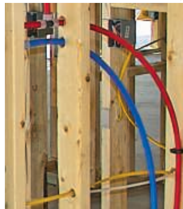
FIGURE 3. Hypertherm 2399 resin for domestic and commercial hot-and-cold water plumbing enhances the flexibility of plastic pipe so installers can bend water lines at turning joints, allowing for ease of installation.
