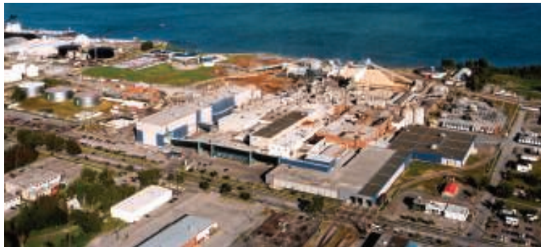
FIGURE 3. Shown here is the pulp-and-paper mill in Trois Rivières, Quebec. A demonstration plant for producing a type of nanocellulose material was recently built at the mill
